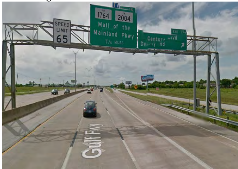
Figure B.55. HOU-16-2 - Asphalt pavement. (Source: Google)
