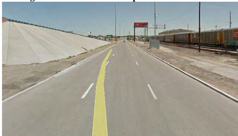
Figure B.15. ELP-06-2 – TxDOT Roughness Data Collection.
