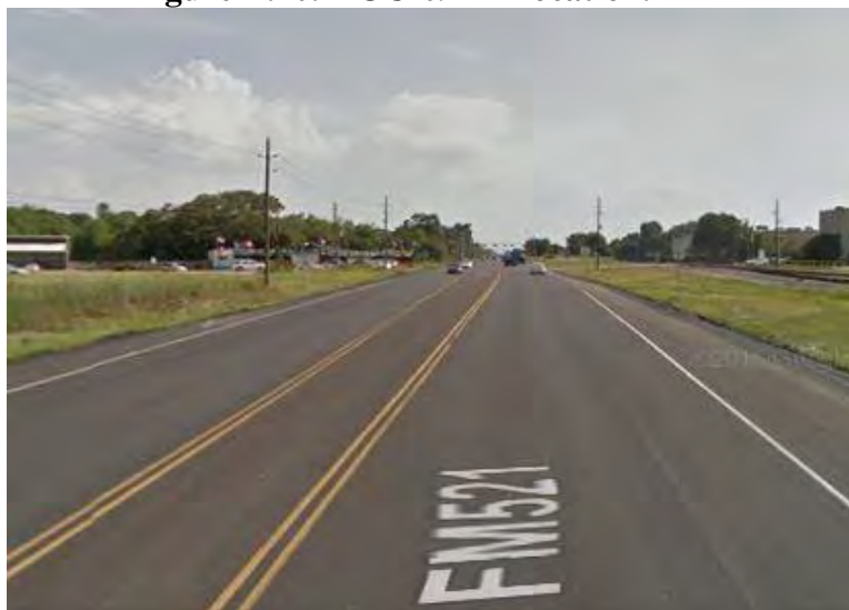
Figure B.41. HOU-09-2 - Asphalt pavement. (Source: Google)
