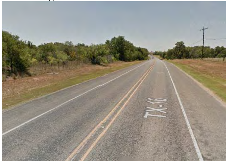
Figure B.73. SA-01-2: Concrete pavement. (source: Google earth)
