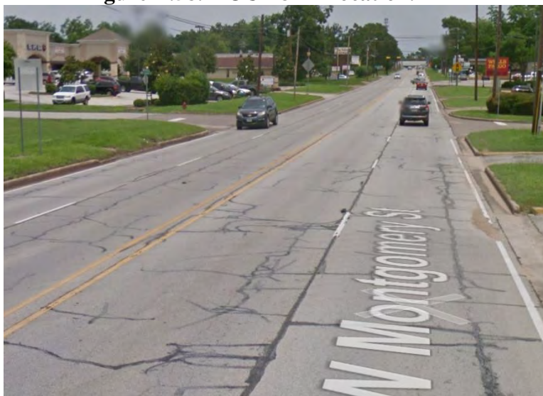
Figure B.59. HOU-18-2 - Asphalt pavement. (Source: Google)
