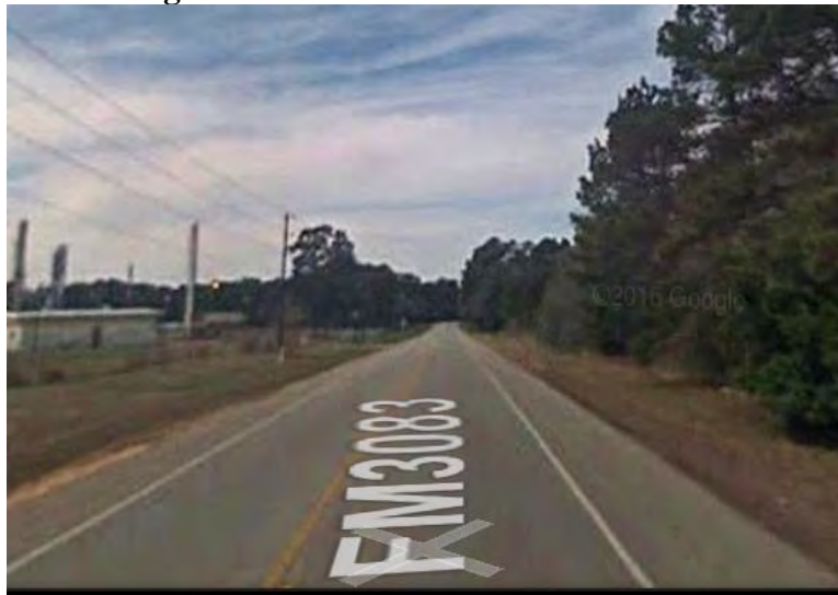
Figure B.57. HOU-17-2 - Asphalt pavement. (Source: Google)
