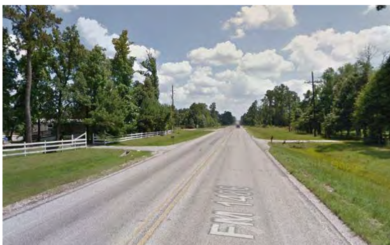
Figure B.31. HOU-04-2 - Asphalt pavement. (Source: Google)
