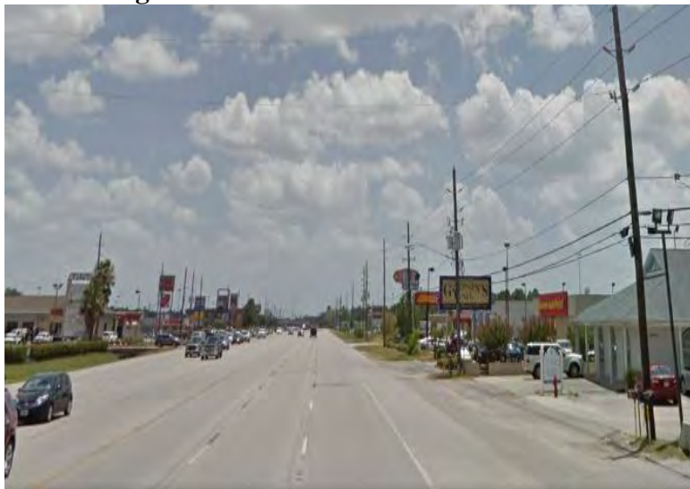
Figure B.67. HOU-23-2 - Asphalt pavement. (Source: Google)
