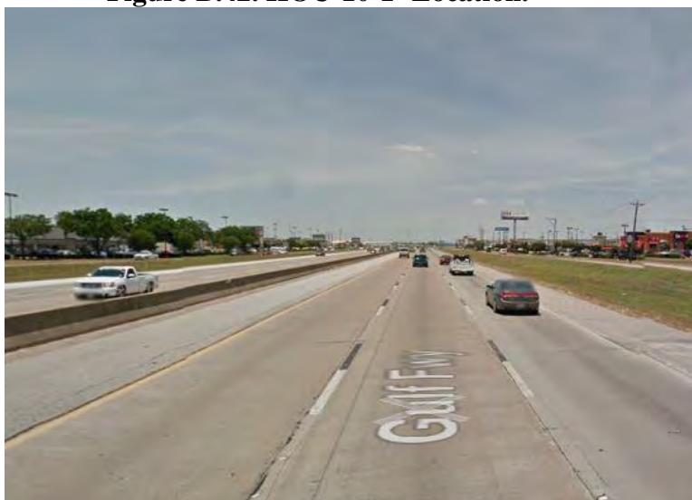
Figure B.43. HOU-10-2 - Asphalt pavement. (Source: Google)
