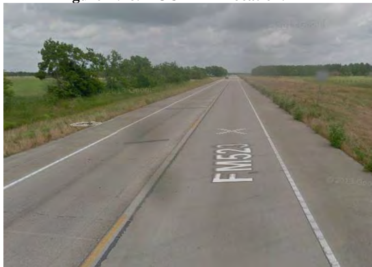
Figure B.47. HOU-12-2 - Asphalt pavement. (Source: Google)
