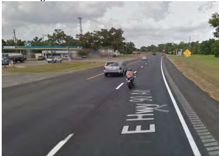
Figure B.37. HOU-07-2 - Asphalt pavement. (Source: Google)
