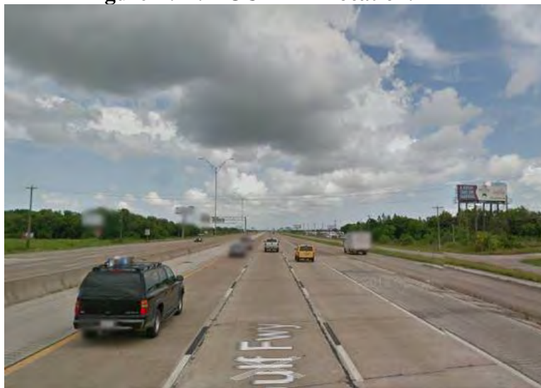
Figure B.45. HOU-11-2 - Asphalt pavement. (Source: Google)
