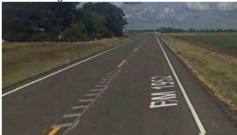
Figure B.27. HOU-02-2 - Asphalt pavement. (Source: Google)
