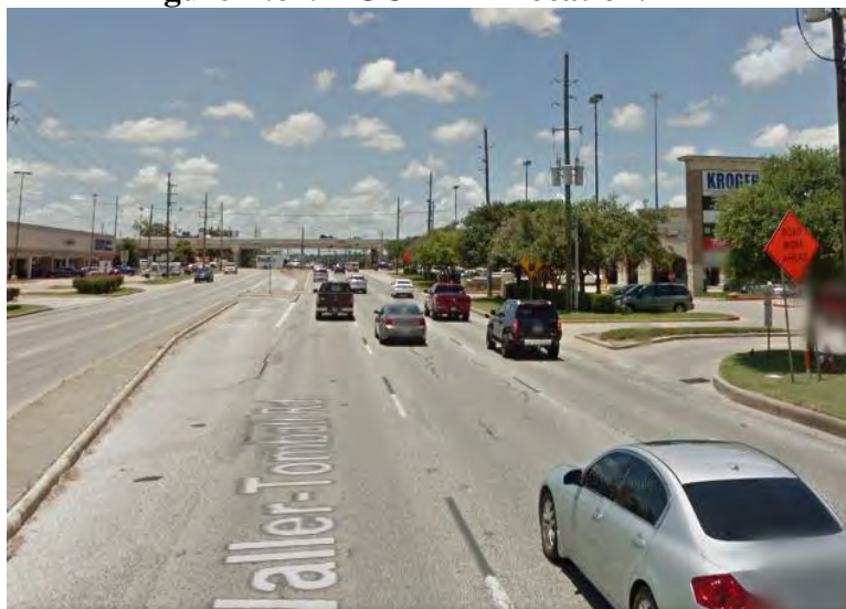
Figure B.65. HOU-22-2 - Asphalt pavement. (Source: Google)
