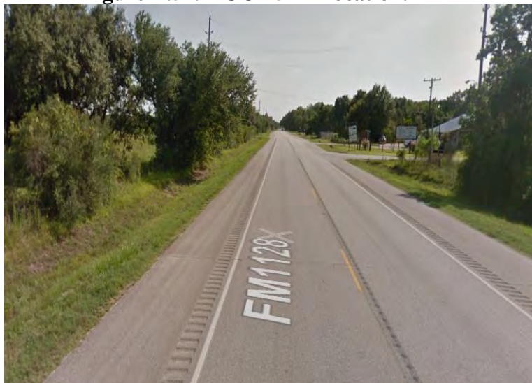
Figure B.53. HOU-15-2 - Asphalt pavement. (Source: Google)
