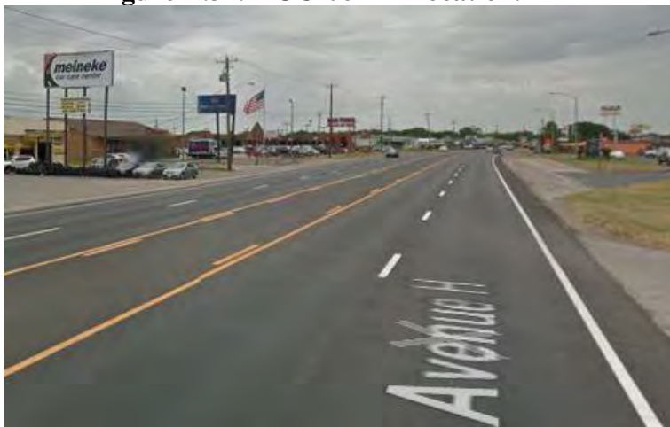
Figure B.35. HOU-06-2 - Asphalt pavement. (Source: Google)
