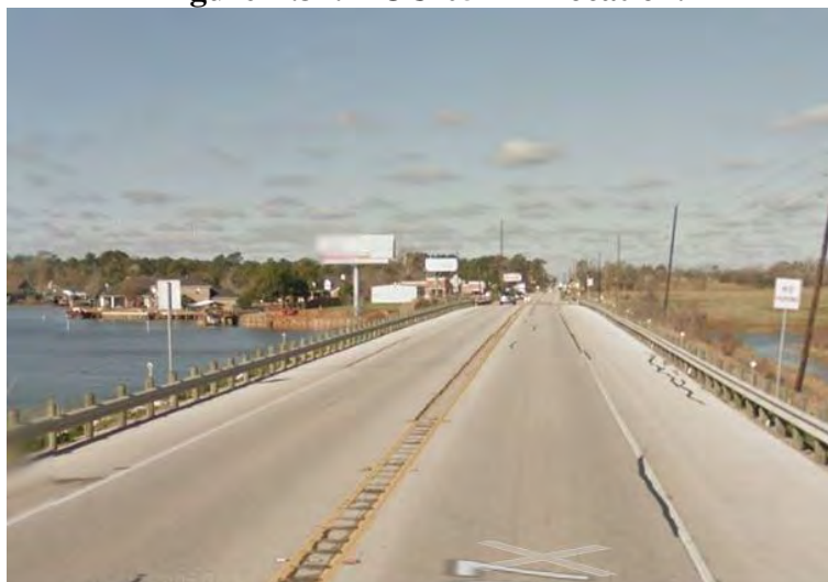
Figure B.33. HOU-05-2 - Asphalt pavement. (Source: Google)
