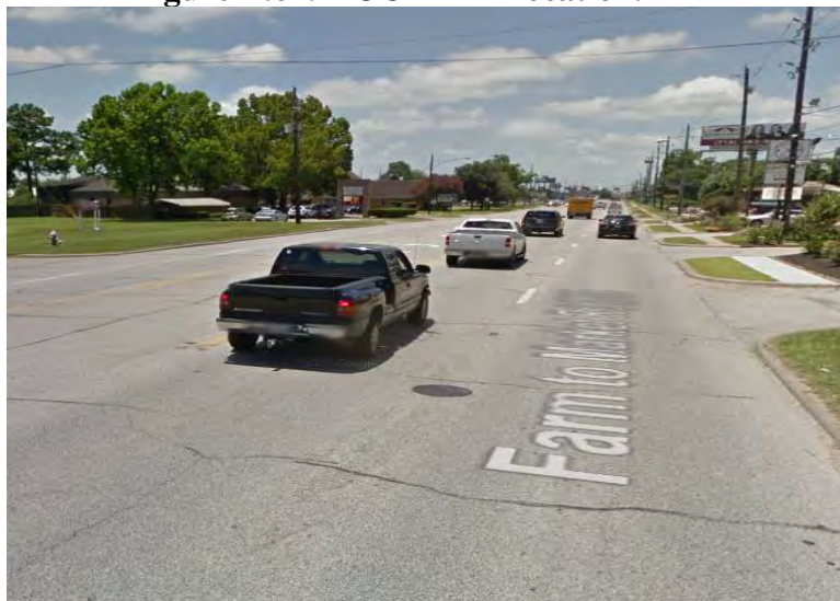
Figure B.63. HOU-21-2 - Asphalt pavement. (Source: Google)
