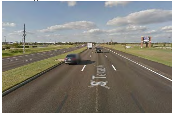
Figure B.25. HOU-01-2 - Asphalt pavement. (Source: Google)
